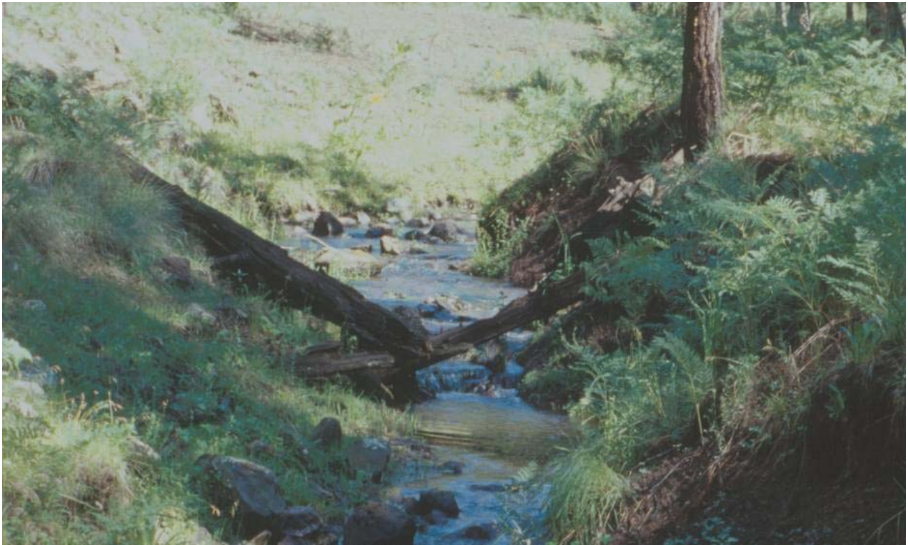
Figure 4: View of Soldier Creek before placement of riffle formation, June 1998. The logs in the channel were remnants of a failed grade control structure dating to the 1980s.
