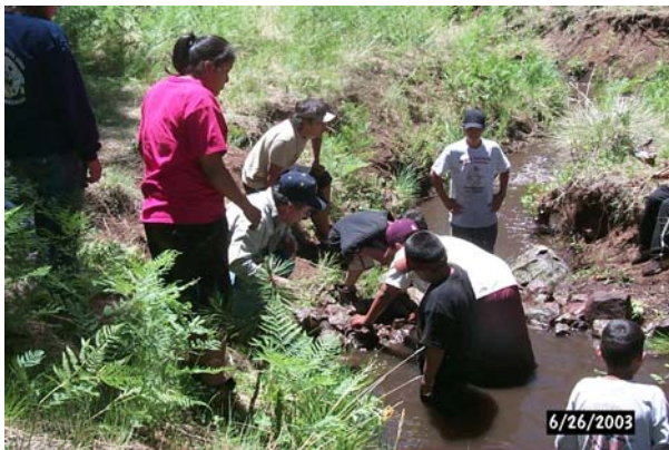
Figure 3: Participants at the White Mountain Apache Tribe’s summer youth camp helped to build riffle formations by hand using rocks from adjacent side-slopes.
